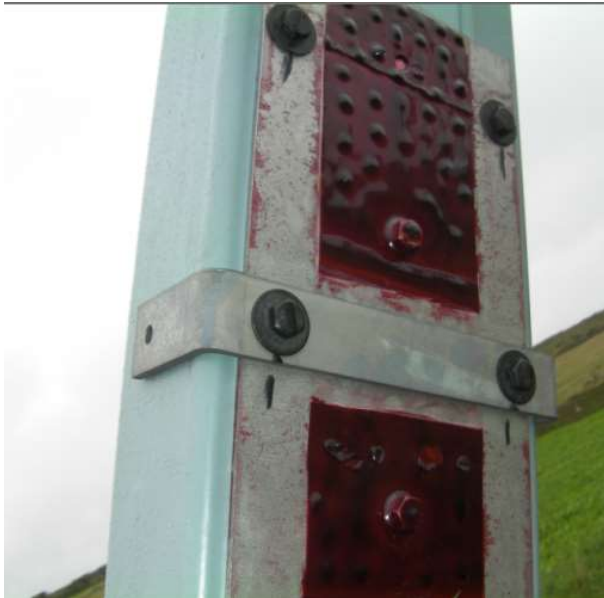
Figure 6.2 Brake Coils and Rear Cover Boom Bracket fitted to tail booms
