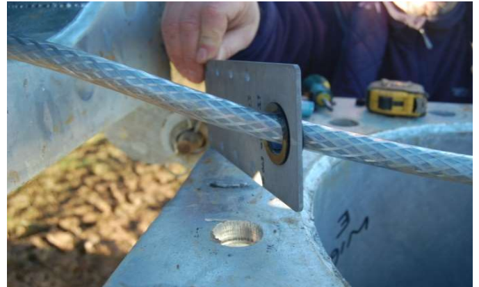
Figure .2 Fitment of Cable Guide bracket
