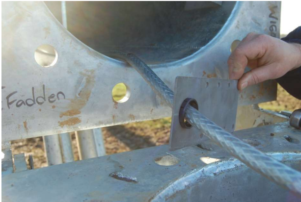
Figure .2 Fitment of Cable Guide bracket
