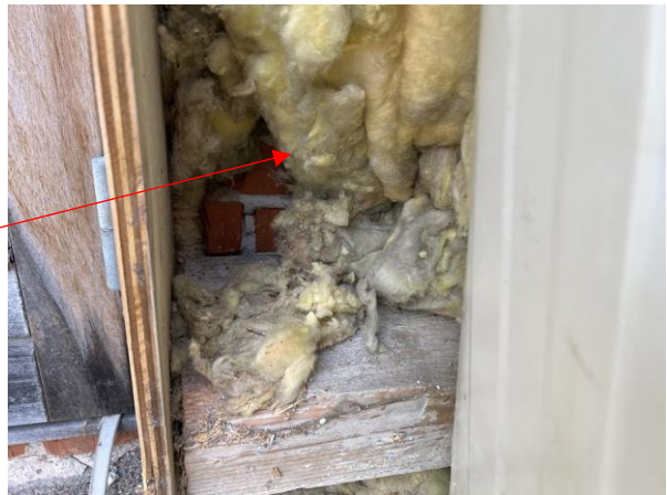
#4 Ca. 300 mm glasuld bag stålbeklædning.
